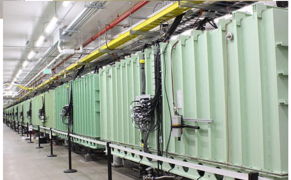
5-cell 644 MHz cavities for FRIB upgrade
